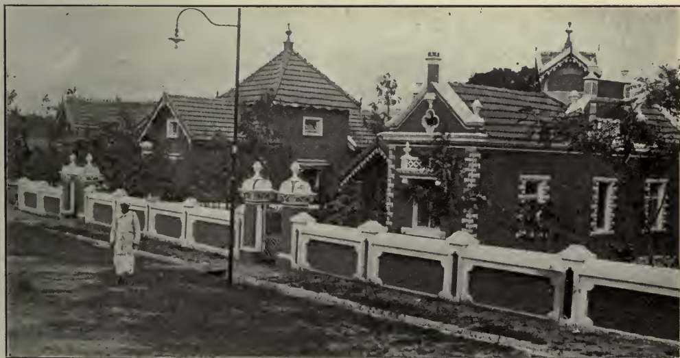
TWO COMPLETED COTTAGES IN FRASER TOWN, WITH THE OWNER
